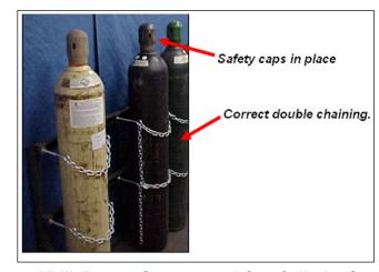
Figure VI-III. Proper Compressed Gas Cylinder Storage
